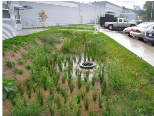
Rainwater Harvesting through use of Rain Garden
