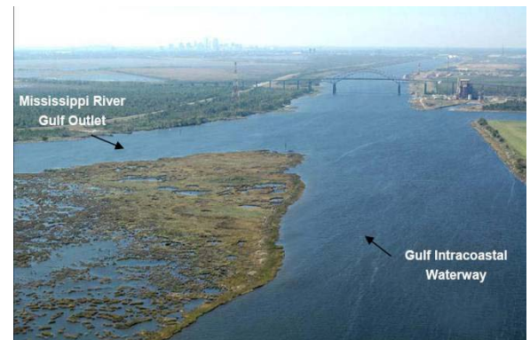
Aerial view of Inner Harbor Navigation Canal Project
