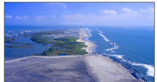
Engineered barrier islands have been successful in the region
