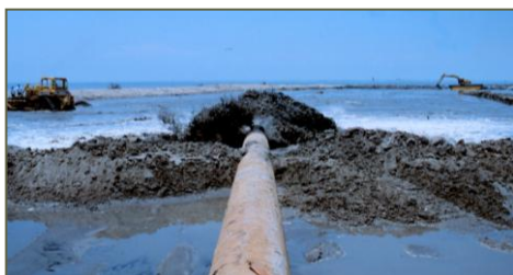
Pumping dredged sediment to form land is cost-effective
