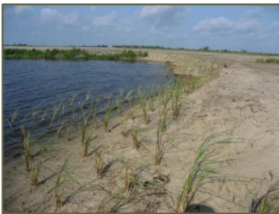
Marsh planting on dredged sediment fill
