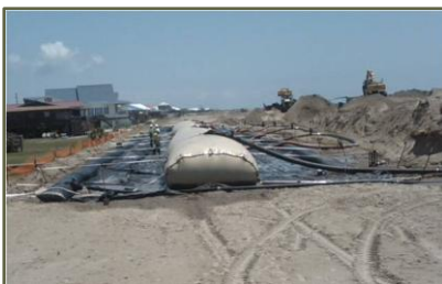
Sand-filled construction fabric geotube installed for dune strengthening
