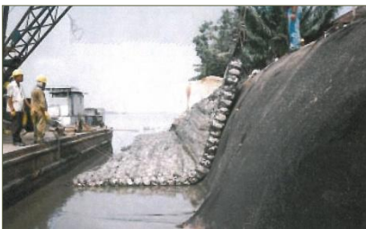
Chamber revetment employed in high energy area
