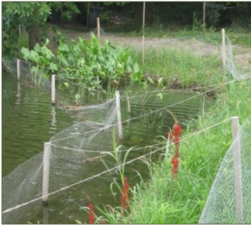
Shoreline stabilization and emerging wetland creation
