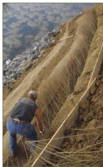
Dormant native vegetation installed between lifts of carefully compacted soil
