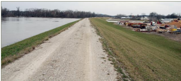
Standard uniform turf levee
