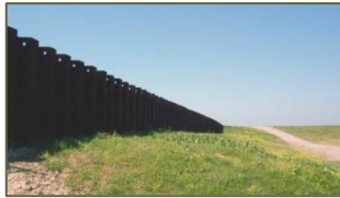
Plaquemine's Parish – Five Floodwalls
