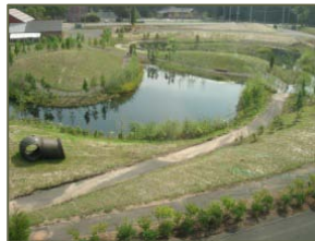
South Central Connecticut Water Treatment Plant
